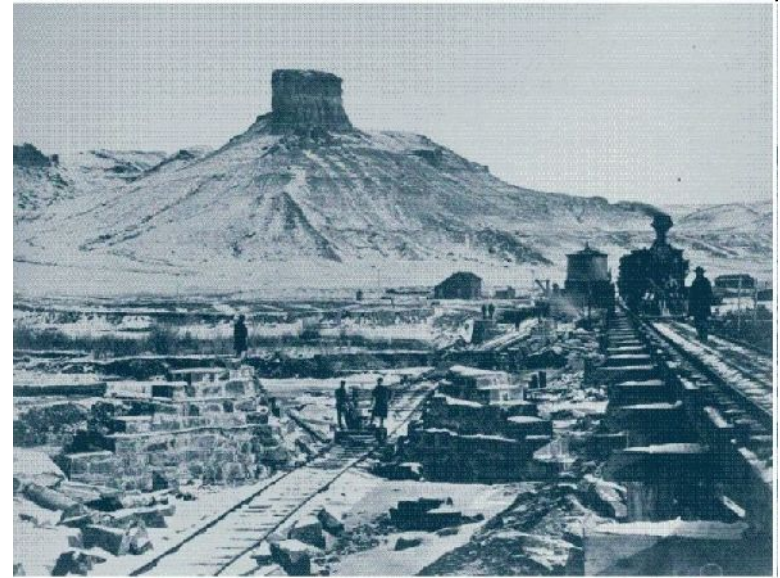
Andrew J. Russell Railway construction in the Green River Valley, Wyoming, near Citadel Rock, 1868. Albumen print
